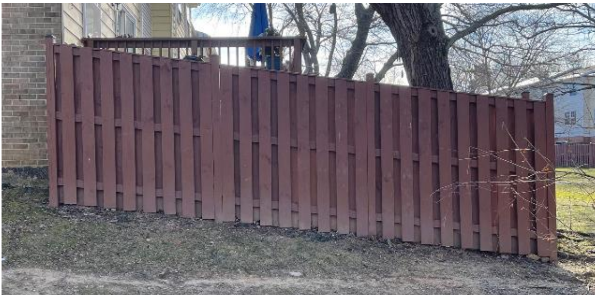
Fence Construction on Hill – Sloped
