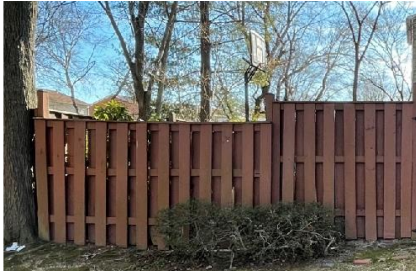
Fence Construction on Hill – Stepped
